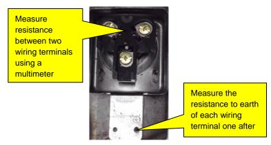
Measure the resistance to earth of each wiring terminal. The value should be 10 M $\Omega$ . If not, the compressor has an internal fault.
